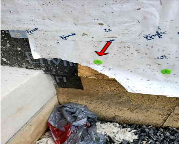
Front elevation near front door
