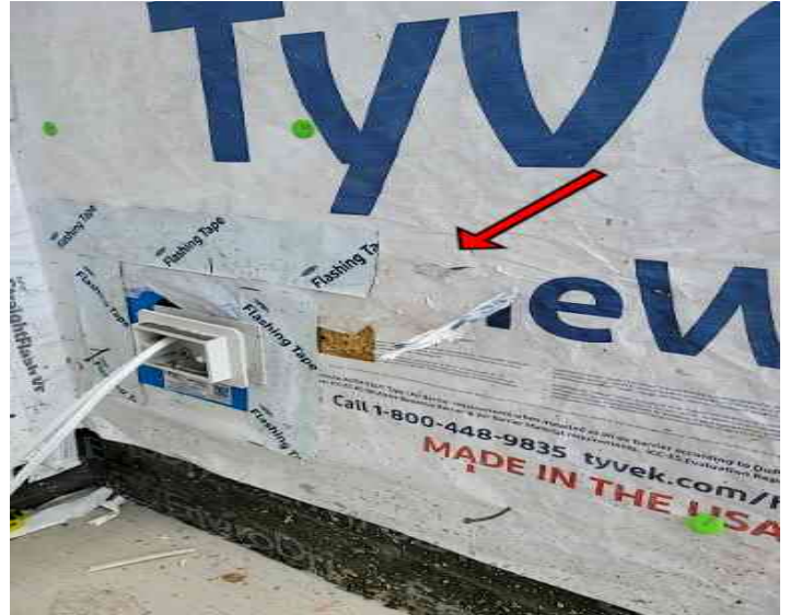
Front elevation near front door.
