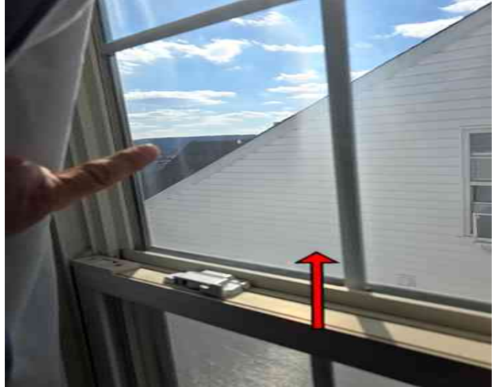
Upper window left side third floor
