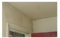
You can investigate any soft spots on the first floor by looking in the basement or crawlspace. Soft spots on the second floor are most likely due to plumbing, roof or wall leaks. Some exterior products such as manmade stucco is known for trapping moisture.
