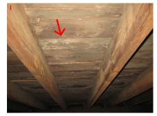
Attics can collect moisture. The source is often from bathroom vents deposited into the attic space with too little ventilation. Do some scouting. How does the sheathing look, is it black or moldy? Is there an odor? Do you see vents? Is the insulation blocking the vents? Do bathroom fans vent here?
