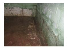
Check for moisture signs such as standing water in your basement, black or white stains on the foundation walls, or discolorations on the sub-floor or framing. Identify the locations of the bathroom and kitchen, and look from below for leaks and stains in the basement or crawlspace. These are all signs of excessive moisture.
