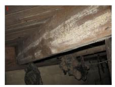
Temperature changes will cause the moisture trapped in warm air to condense on cooler surfaces. If left wet for 24 to 48 hours, you will end up with mold, rot and foul odors.
