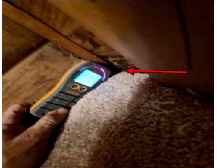
Wet stain noted middle rear bedroom
