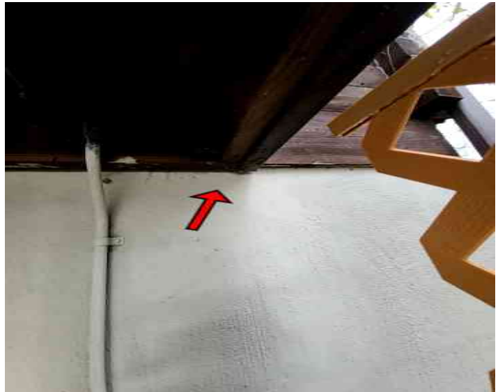
Poorly connected framing noted at deck
