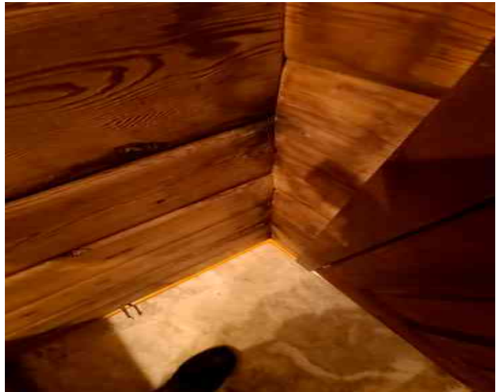
Stains in master bath not wet at time of inspection
