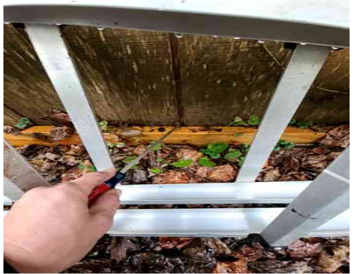
Some visible rot above trim board..
