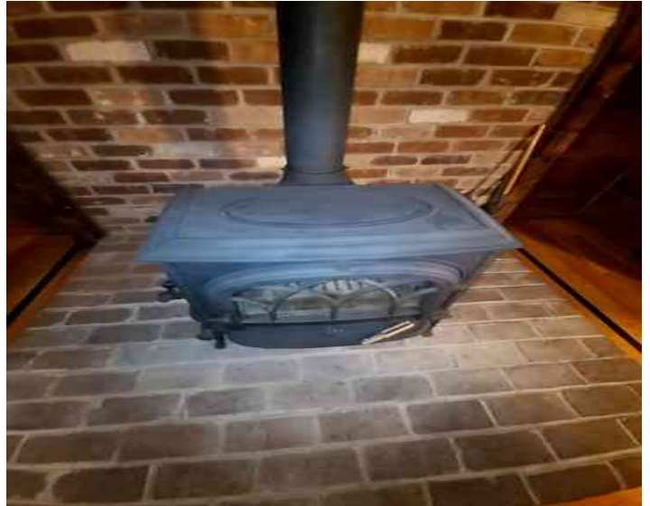
Second wood stove excluded from inspection also
