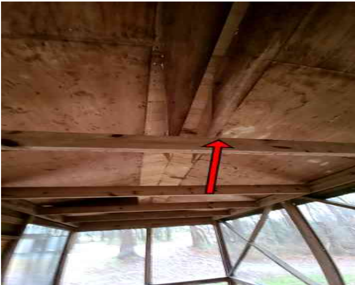
Delamination noted in pavilion ceiling and should be repaired
