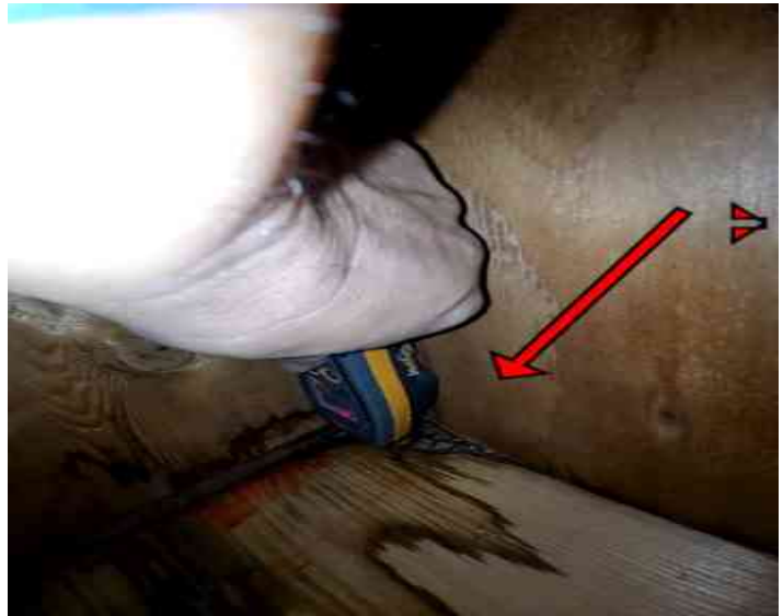
Center of rear wall
