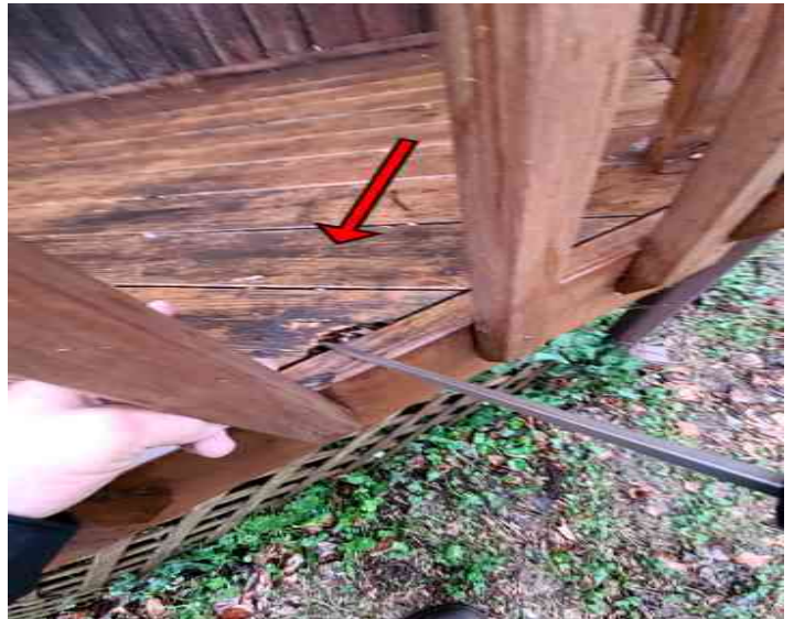
Rot at front deck should be repaired.
