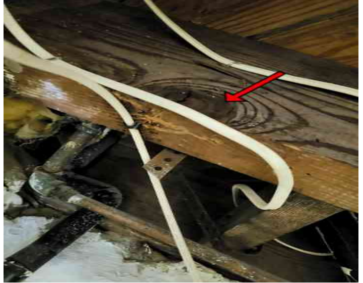
Termite damage noted floor joist near heating equipment
