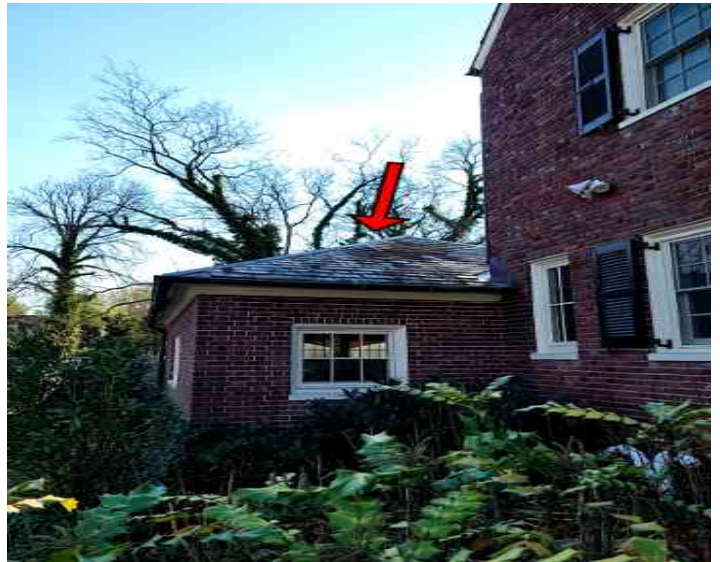
Asphalt patch on roof system over garage
