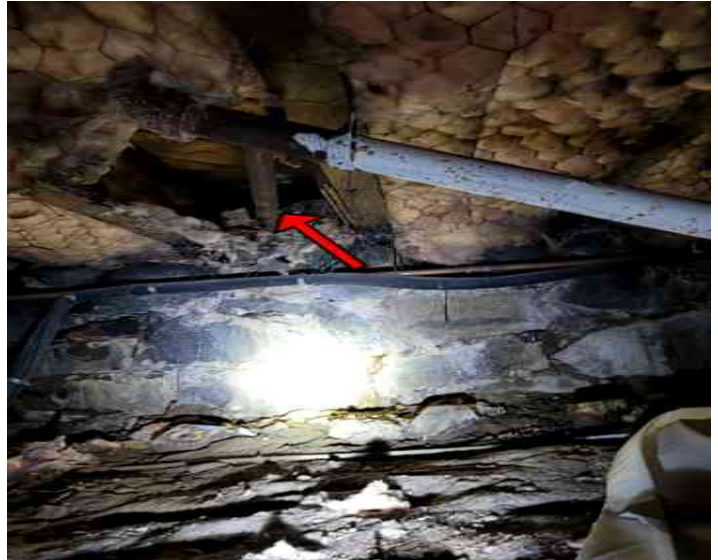
Insulation limits inspection in crawl space
