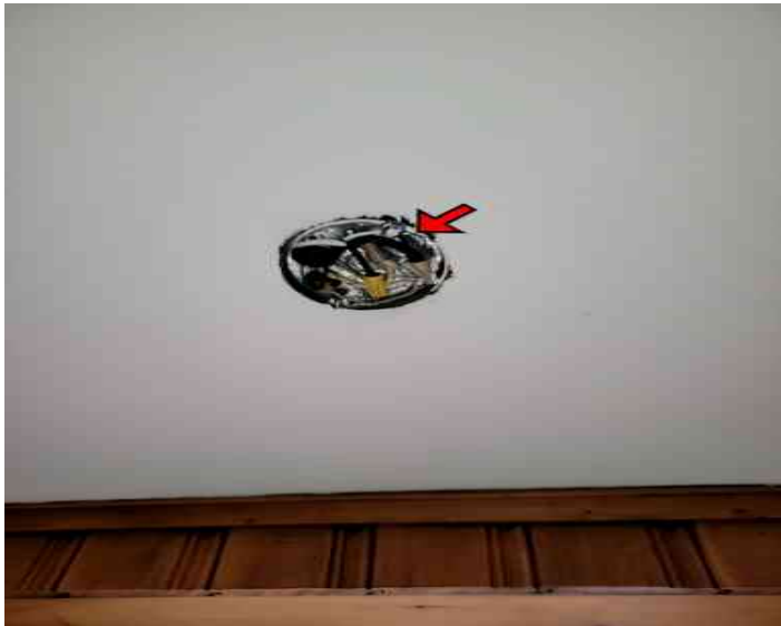
Missing light fixture at the 2nd floor hallway and should be repaired.
