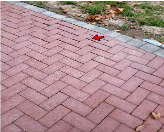
Loose brick at the rear and should be repaired.
