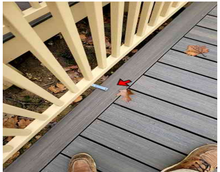
Missing screws at the railing bracket and should be repaired.
