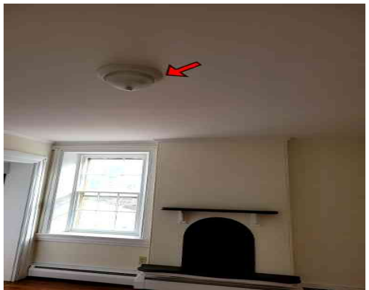
2nd floor middle bedroom light did not work when tested and should be evaluated and repaired
