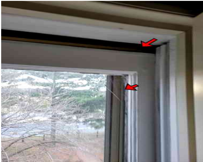
3rd floor front bedroom left window has cracked glass and does not close properly and should be repaired.
