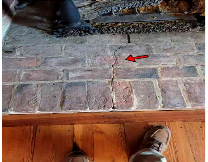
Cracks at the hearth was noted.
