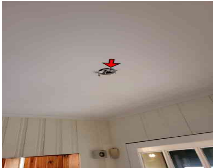
Missing light fixture was noted at the side porch entryway and should be repaired.
