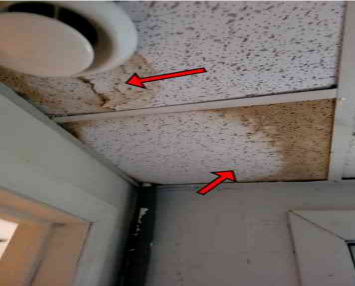
Water damaged tiles noted
