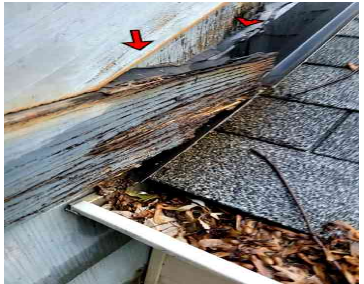
Rotted areas should be replaced
