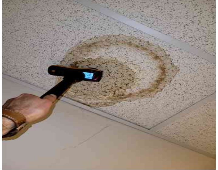
1st floor bathroom.
