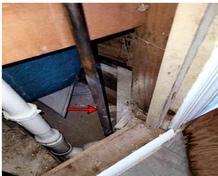
Apartment 2 access panel
